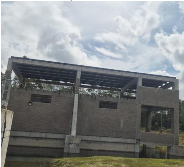
Edificio RAS – WAS
