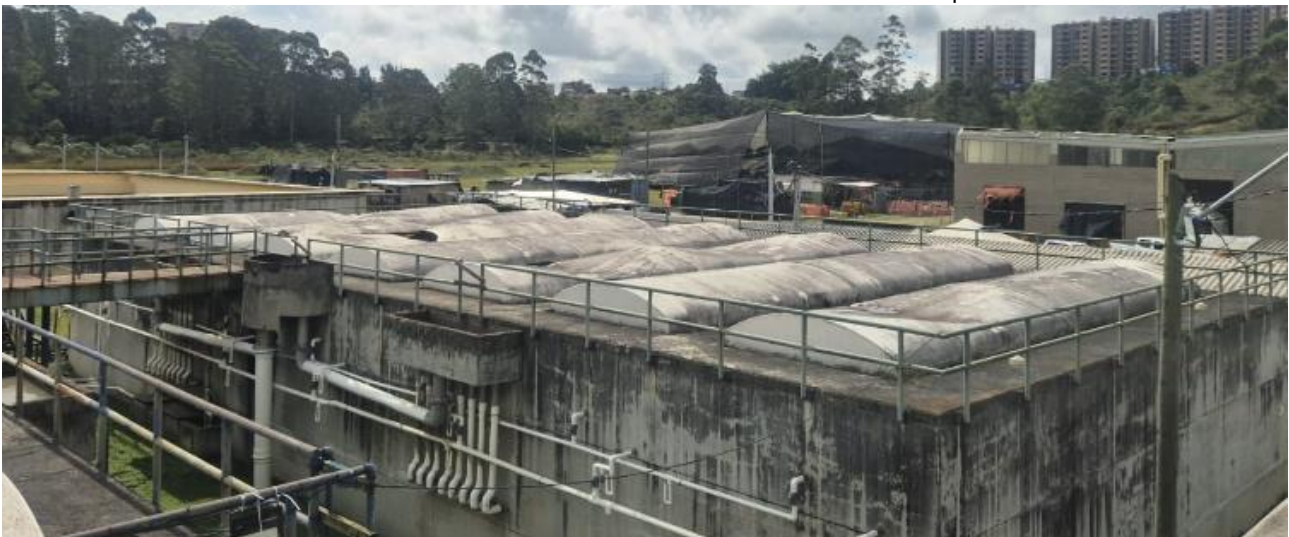
Reactor UASB
