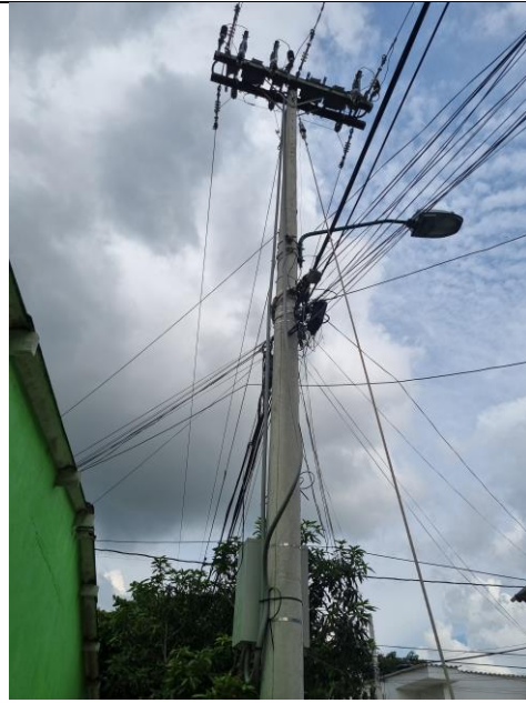
10°54'41.3"N 74°47'07.2"W, Estructura final tramo 4, 110 ml
