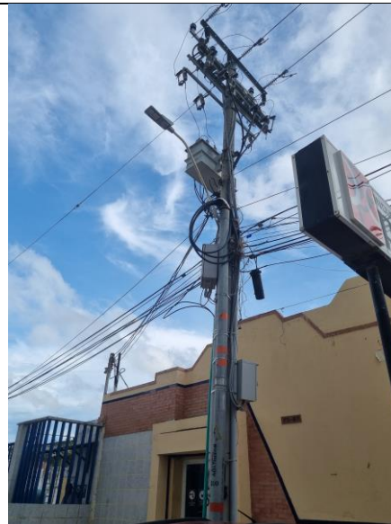
11°00'44.0"N 74°47'40.4"W, Estructura final tramo 1 cable 4/0 340 ml.
