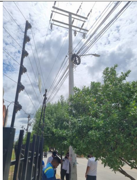
10°55'00.7"N 74°46'54.5"W, finaliza tramo 1 conductor AAAC 123.
