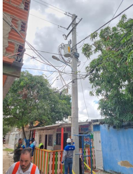
10°54'43.1"N 74°47'03.4"W, Estructura final tramo 3 conductor AAAC 123, 411 metros
