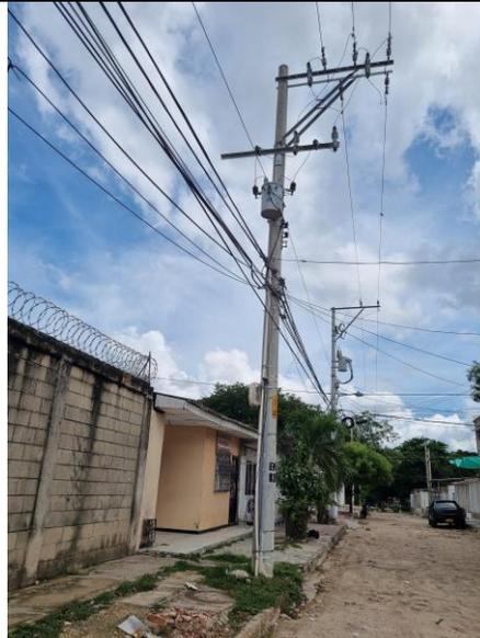
10°54'22.0"N 74°46'56.3"W, Estructura final tramo 1 cable AAAC 123, 300 ml.
