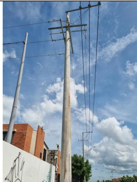
10°55'10.9"N 74°46'56.4"W, Estructura fin de tramo 2 conductor AAAC 123, 300 ml.
