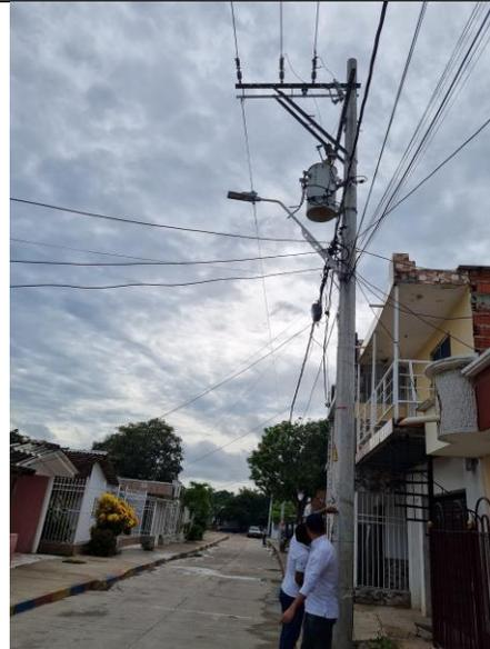
10°59'23.0"N 74°46'38.6"W, Estructura final tramo 1 cable AAAC 246,9 80 ml.
