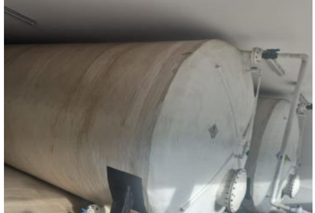
Tanque coagulante
