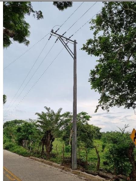
8°57'07.0"N 75°27'10.3"W Estructura final AAC 123
